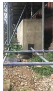
The temporary works structure was ballasted by concrete kentledge blocks, buried up to 2m in the ground
